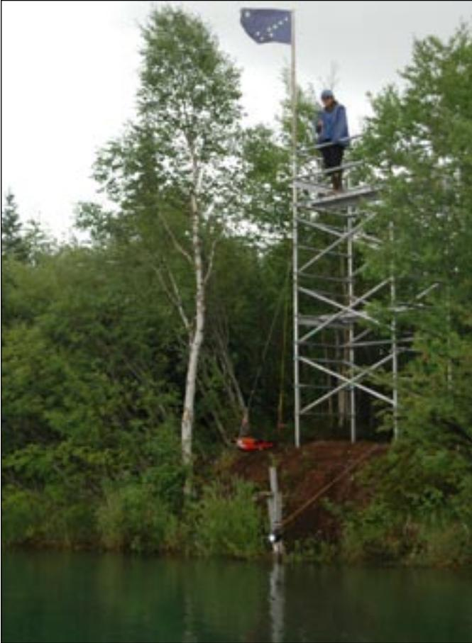
**FIGURE 1.** — Example of a counting tower used on the Newhalen River, Bristol Bay, Alaska. This tower is constructed of lightweight aluminum scaffold and is stabilized with guy wires. Here, Libby Baney conducts a 10-minute systematic count.
