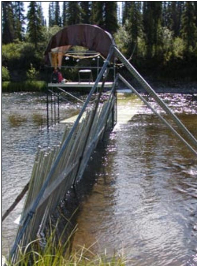
**FIGURE 8.** — Example of a diversion weir used in a counting tower project to guide fish into observable range. (Photo courtesy of the Alaska Dept. of Fish and Game.)
