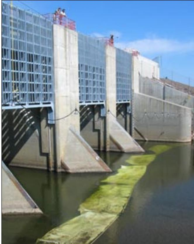
**FIGURE 2.**— Example of a counting tower “surrogate” used to estimate escapement on the Chena River, Alaska. Biologists conduct counts from the closest piling. Note contrasting substrate panels that improves visibility of migrating fish. (Photo by the Alaska Department of Fish and Game.)
